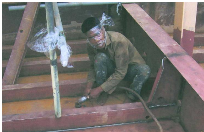
External engineer using dangerously inappropriate protection equipment
